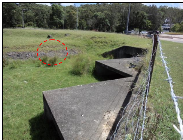
Figure 18: Photo showing both sets of culverts that discharge under Wyong Road/Tonkiss Street intersection. (Red circle identifies location of the northern culverts).
